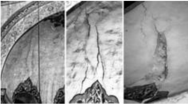
Figure 17. Damage of the earthquake 1999 (right), same situation 1979 (middle) and earlier than 1908 (left)
