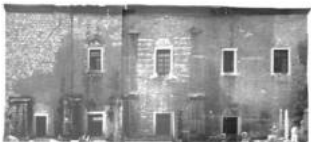
Figure 6. North side of KAM
