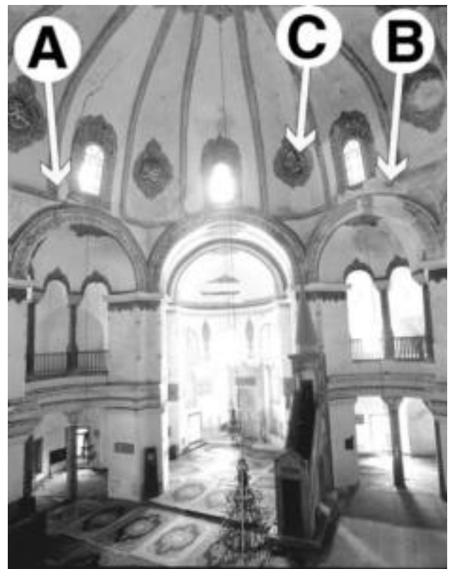
Figure 7. Location of the discussed cracks
