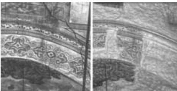
Figure 9. Crack (B): left: in the year 1968 right: in the year 2000
