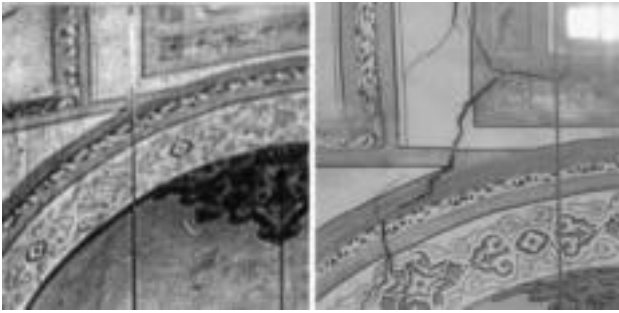
Figure 8. Crack (A): left: before 1908 right: in the year 2002
