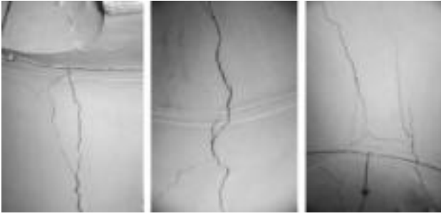
Figure 16. Damages of the earthquake in august, 1999
