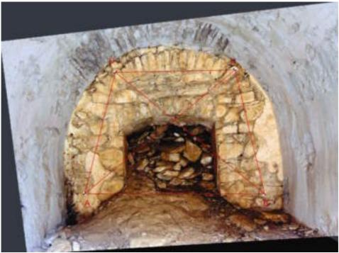
One example of the photogrammetric restitution of a wall.
