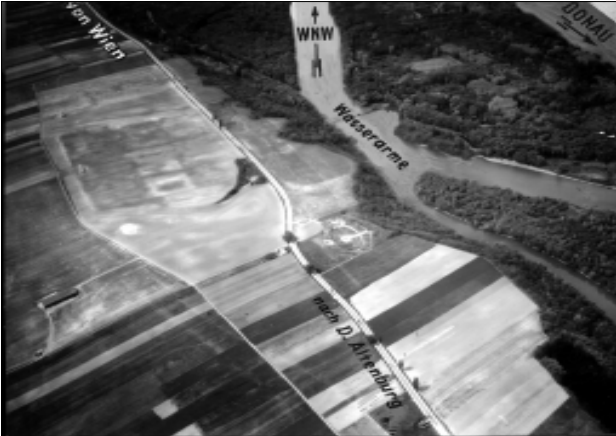
Figure 3: Oblique photograph from the 28 th of April 1939 showing the Roman military camp. The enclosure walls and the system of the inner buildings can be seen clearly.
