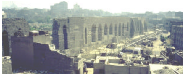
Figure 2. Overall view of the Aqueduct
