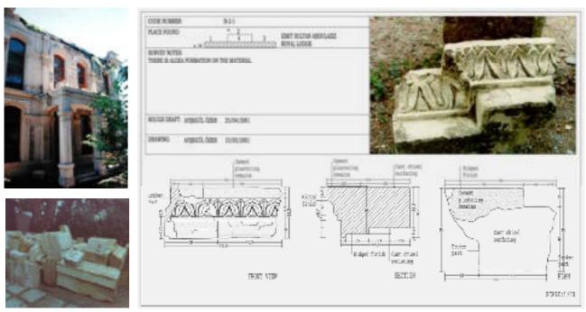
Figure 6a, 6b, 6c. The view of the east facade with collapsed debris of the cornice at roof level parapet and collected fallen pieces in the garden which were classified, numbered and then documented in 1:10 scale detail.
