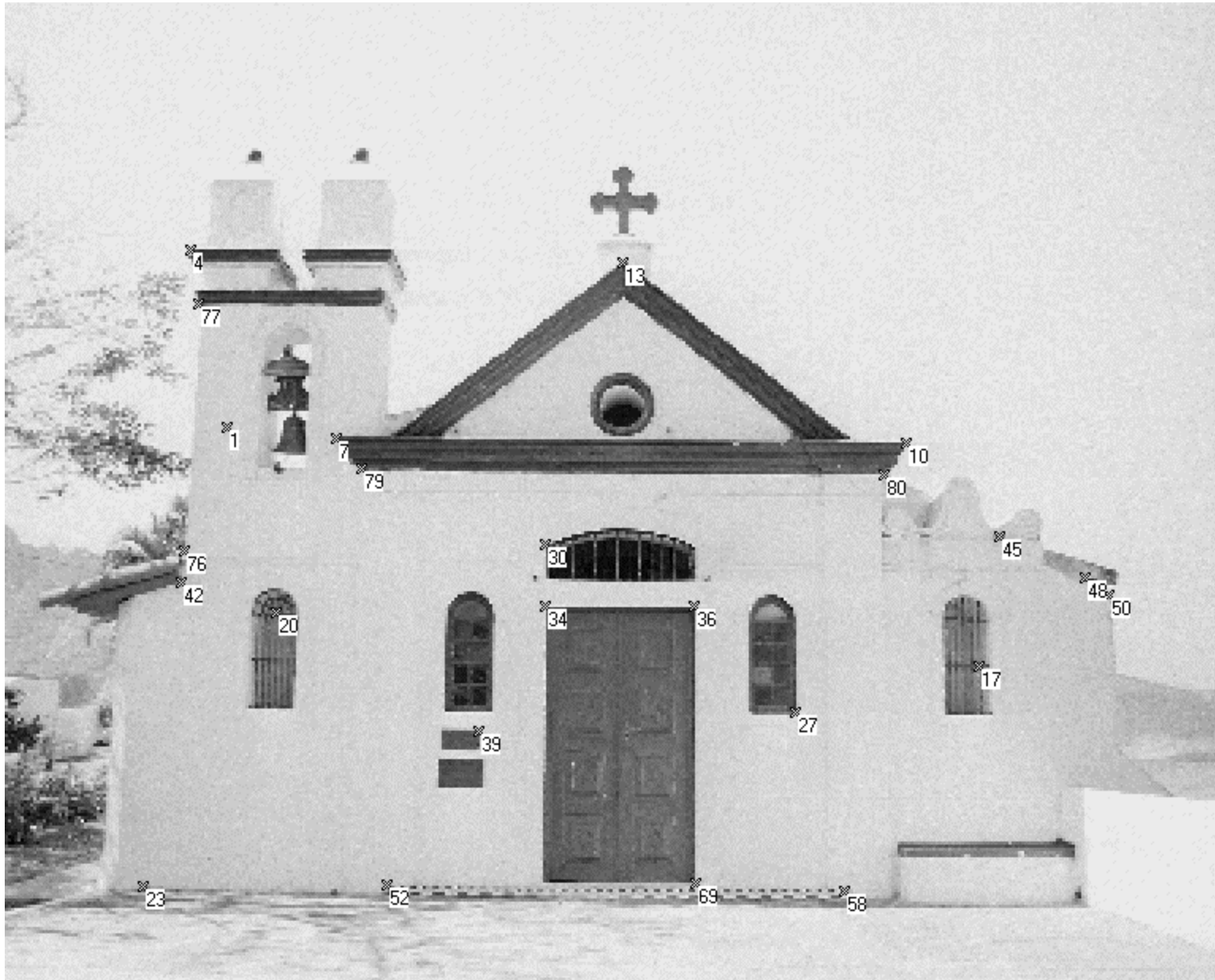
Fig. 3 - Photograph of the principal façade of the Chapel with control points indicated
