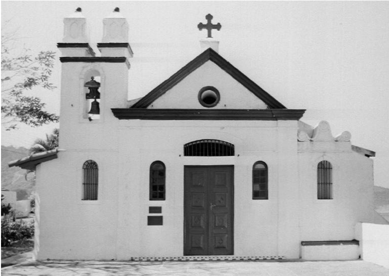
Fig. 2 - Reduced ortophoto of the principal façade of Santa Bárbara Chapel , Santa Cruz Fortress - approximate scale 1:50
