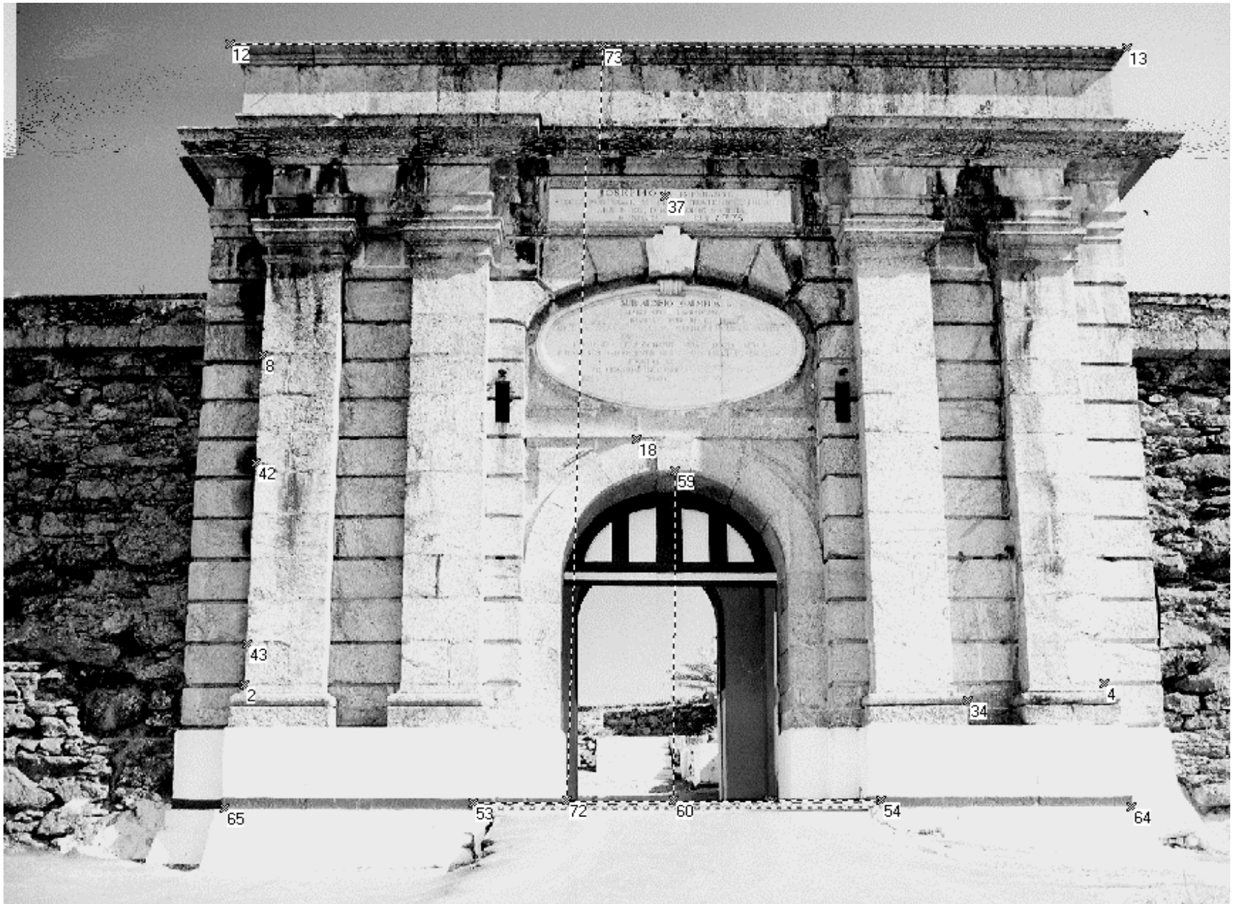
Fig. 5 - Main Entrance of São Luiz Fort with control points indicated
