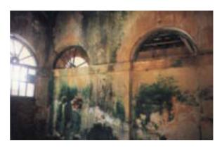
Figure 5. Wall surface covered with fungal and mosses.
