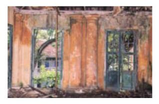
Figure 6. The upstairs building condition, timber door was rotten and damage. The columns were mostly effected with rising damp and crumbling plaster problems.
