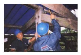
Figure 9. The Inspection of roof structure
