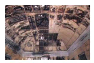
Figure 3. Ceiling board was damaged cause by water penetration through leaking roof.
