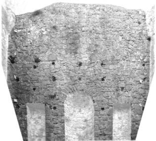
Fig. 5: Digital Rectified Image derived during the field campaign from Fig. 4. The areas outside the rectification plan are shown brighter.
