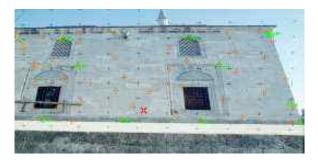
Figure 5. Distribution of control points and tie points for stereo model 1 in northwest facade
