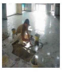
Figure 12: Replacing the broken granite floors.
