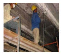
Figure 6: Hacking of the damaged concrete surfaces.
