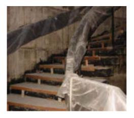
Figure 4: Temporary protection for the spiral staircase
