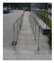
Figure 15: Additional accessible ramp for the disable.
