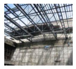
Figure 10: New roof trusses installation
