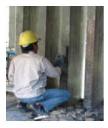
Figure 9: Manual cleaning of soot marks.
