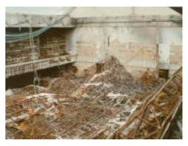
Figure 2: Collapsed roof trusses into the Great Hall
