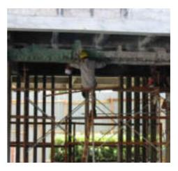
Figure 7: Applying layers of bonding agent Nittobond EP'
