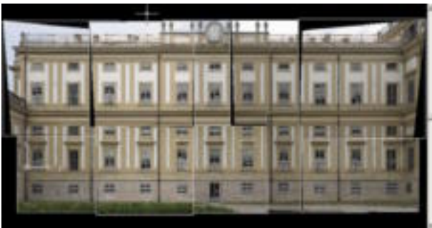
Figure 11. The North annex in AutoCad Map of all the single images straightened before putting them together in the mosaic
