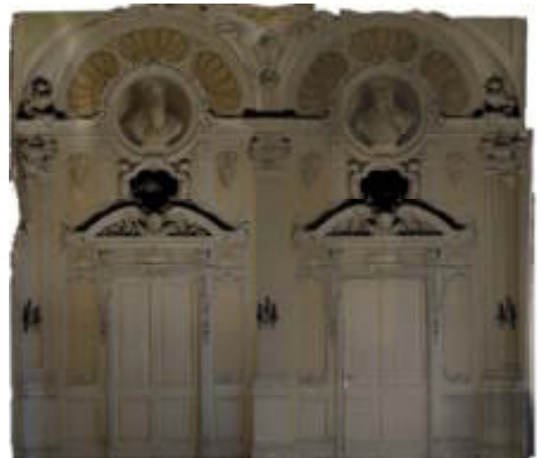
Fig. 4 – The orthophoto of the southern wall.
