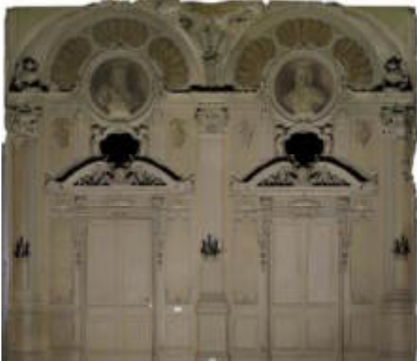
Fig. 6 – The orthophoto of the northern wall.
