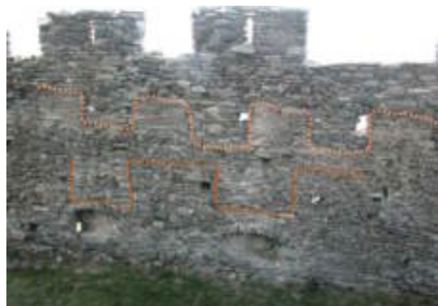
Figure 2. Details of the southern wall
