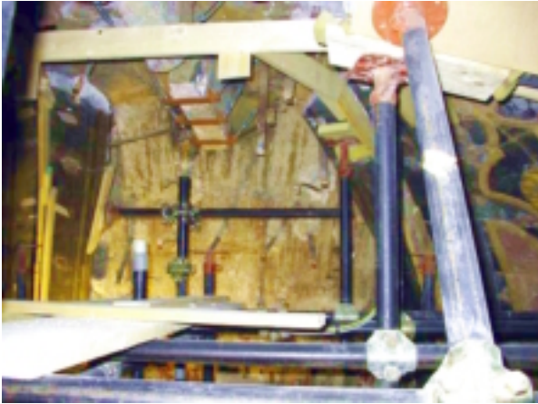
Figure 1. A sliding of the key stone arches as discovered in sector and
