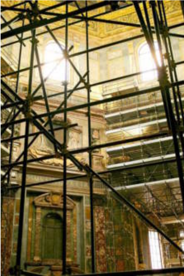
Figure . Scaffolding installations
