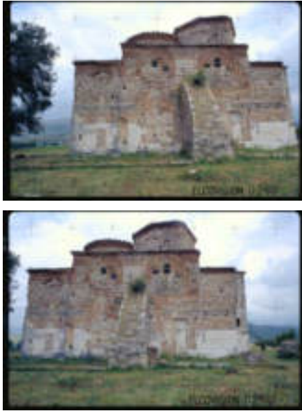
Figure 10. Stereo-pair used for stereoscopic restitution of monastery south facade.
