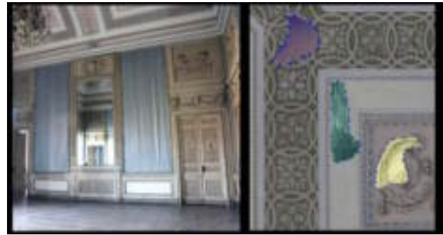
Figure 12 One of the picture of Sala del Trono. To the right the possible mapping of the degradation realized on the orthophoto (NORMAL indications)
