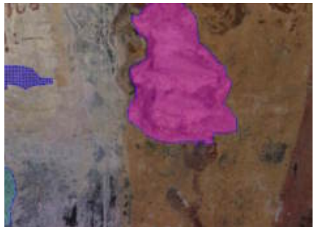
Figure 3. Mapping of decay on a georeferenced digital image
