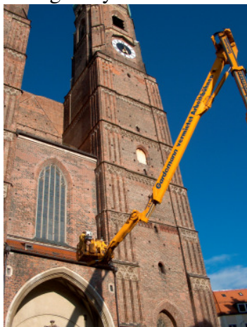
Figure 2: Use of an 83m working platform at the Church of Our Lady in Munich
