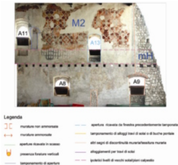
Fig. 1. Example of table showing analysis of internal walls' stratification; south wall, upper floor.
