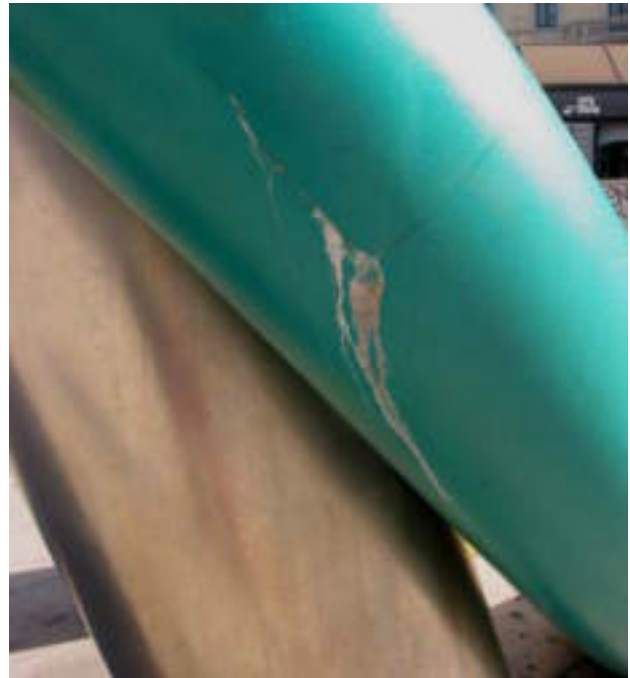
Crevice with drippings
