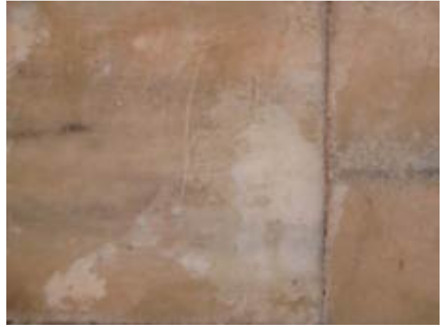
Traces of discoloured synthetic resin
