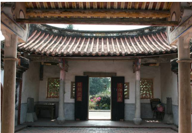
Figure 2. The Front Door of the Yang Ancestral Hall
