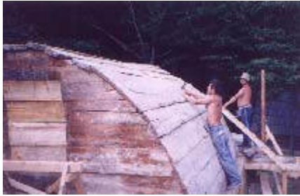
Rebuilding of the vault after the transport
