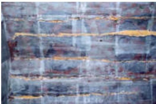
Nave (vault) - strengthening with fish gelatin and thin Japanese paper
