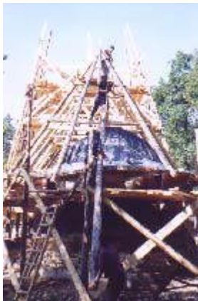
Rebuilding of the roof after the transport
