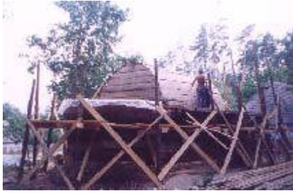
Rebuilding of the vault after the transport
