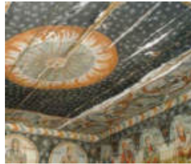
Detail Narthex (wall and ceiling) – before the movement of the church
