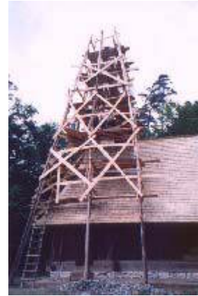
Rebuilding of the spire after the transport
