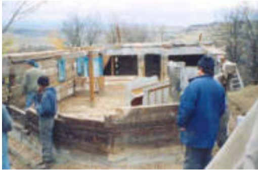
Dismantling of the walls of the church
