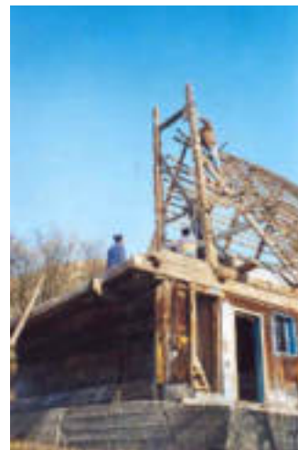
Dismantling of the roof
