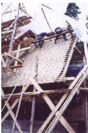
Rebuilding of the roof after the transport
