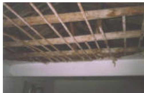
Figure 4. The wooden trusses
