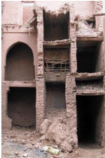
Fig. 4. Casbah in the qsar of Tamnougalt
