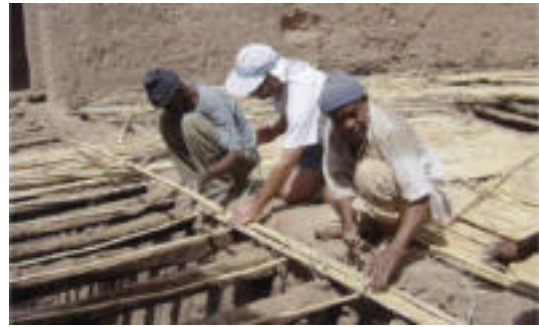
Fig.3. Use of local materials and technologies (Morocco)
