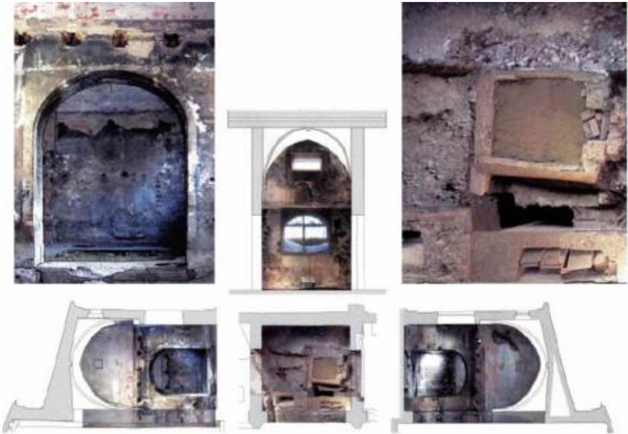
Figure 15. San Francesco al Prato church in Parma, photographical straightening of one chapel
