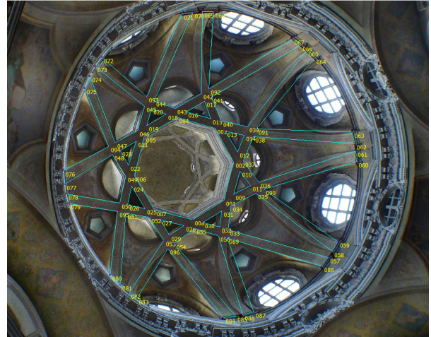
Figure 7 – The ribs of the inner vault of the cupola of San Lorenzo church in Turin, Italy
