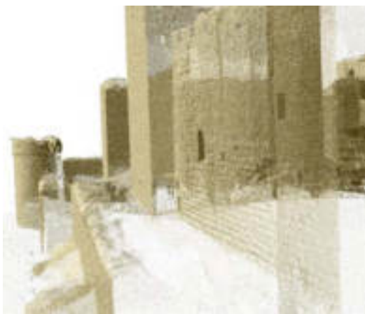
Figure 4: A partial view of walls of the castle with well defined depth planes delimiting spaces for different uses
