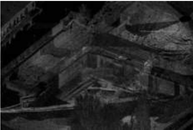
Figure 7. The cloud points: central zone of the dam, 3D view
