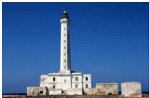
Figure 3. Lighthouse on the island of Sant'Andrea near Gallipoli
