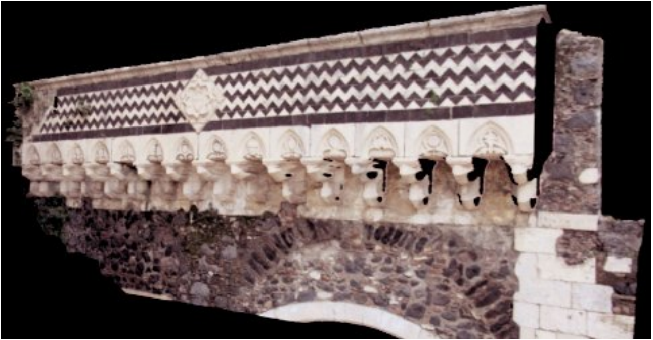
Figure 6. Projection of the photographic image on the mesh
