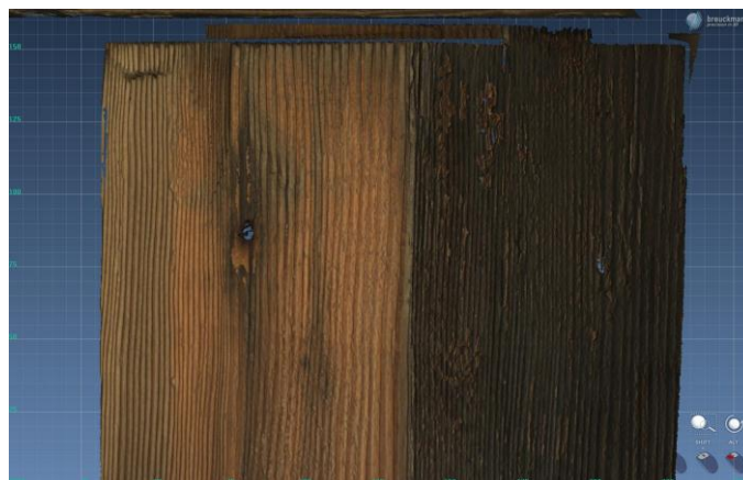
Figure 6: Section of an ablated veranda post from Discovery hut recorded with the smartSCAN 3D -HE. Remnant paint flakes can be seen on the right hand face.
