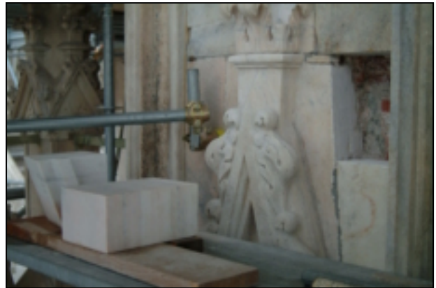
Figure 14. Replacement of a damaged marble block on a counterfort of the Façade during the restoration.
