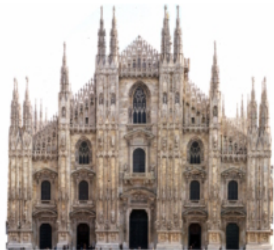
Figure 1. Orthophotograph of the Milan's Cathedral Façade by laser scanning survey.
