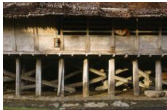
Figure 4: Foundation of a building in North Nias
