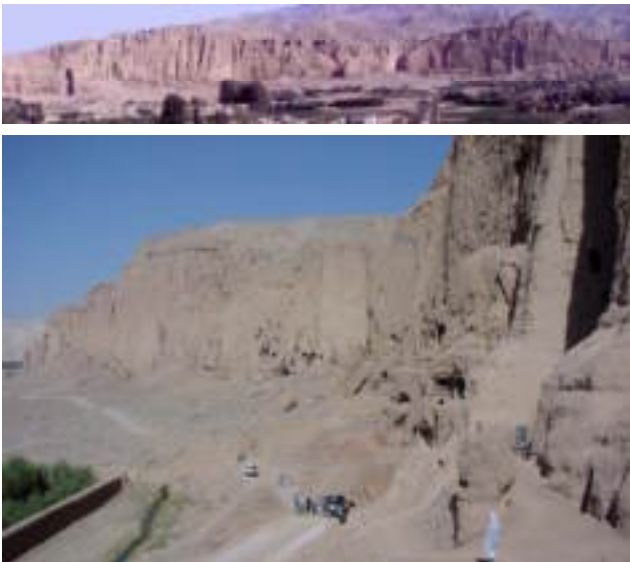
Figure 4: The Bamiyan cliff, approximately 1 km long and 100 m high (above). The cliff as seen from the empty niche of the Small Buddha (below).
