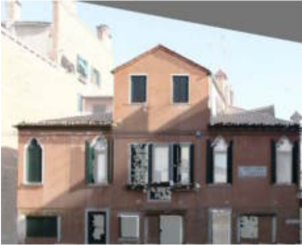
Figure 13. Comparison by overimposition of a photogrammetric rectification and a laser scanner ortophoto
