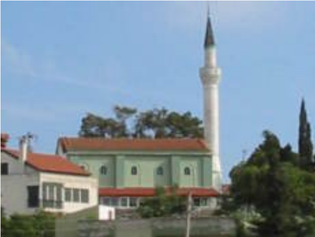
Figure 2. The monument viewed from the north (2005)
