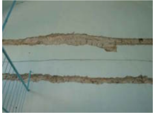
Figure 5. The trace of the central arch of the apse observed at the east wall (2004)
