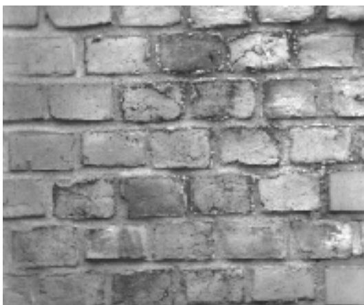
Figure 5. Infrared image acquired with Vidicon-camera (with 850 nm band-pass filter)
