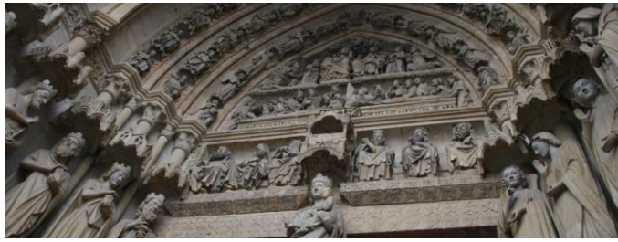
Figure 2: Detail of the southern portal
