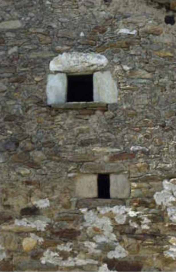
Figure 10. Openings with window jambs and monolithic architraves
