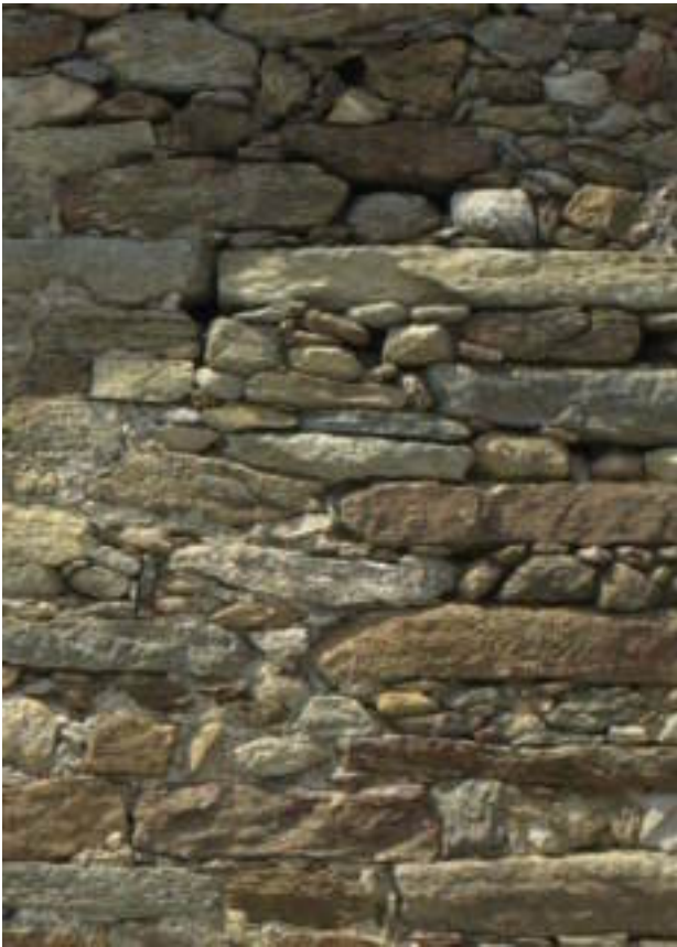
Figure 8. Particular of a building structure's tissue
