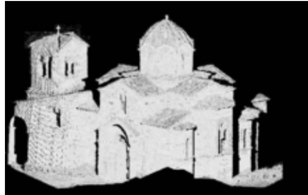
Figure 2. Laser scanning point clouds taken by using the elevator, from south-eastern direction
