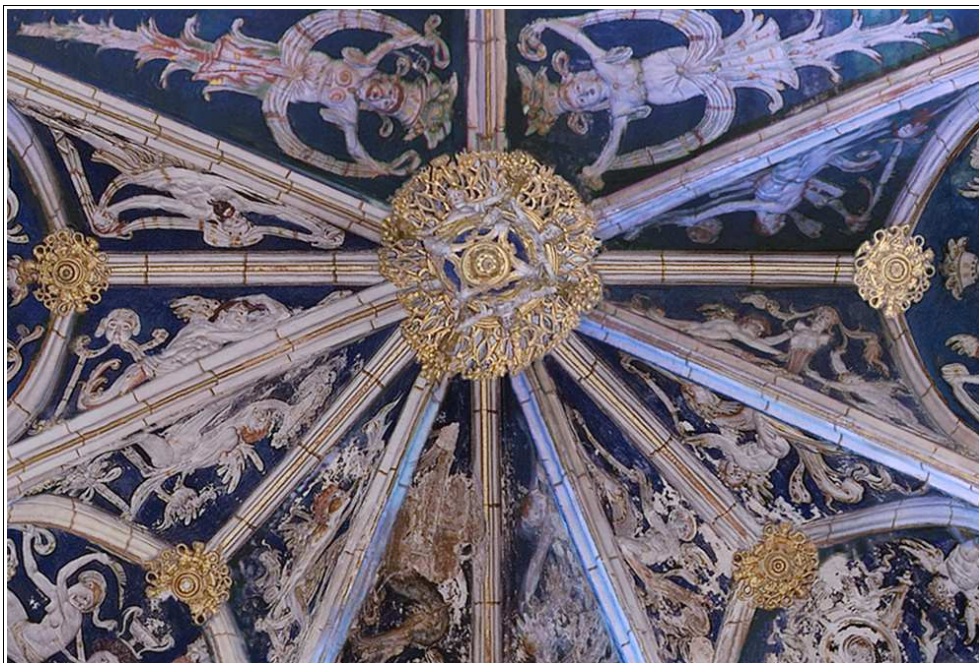
Figure 5: True-orthoimage detail of the vault
