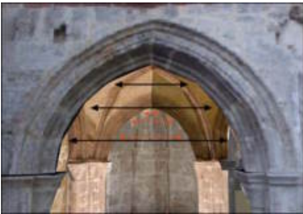
Figure 7: Due to the restriction of planar model faces, real-world curves had to be modelled as polygons. But determining the flexion points manually would have resulted in asymmetric appearances of symmetrical parts of arcs. This could be avoided by intersecting the curved virtual shapes of arcs with horizontal planes.
