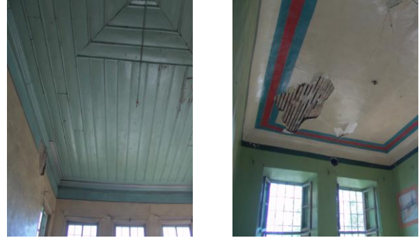
Figure 2. Two flat ceiling from province of Konya, Turkey.
