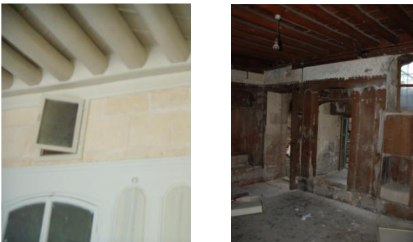
Figure 1. Two inverse ceiling from province of Gaziantep, Turkey.
