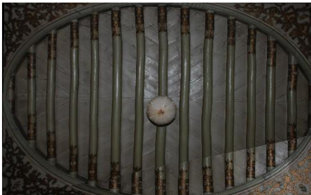
Figure 15. Orthophoto of a ceiling province of Gaziantep, Turkey.
