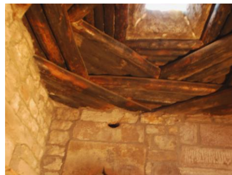
Figure 4. A Corbelled ceiling from province of Kayseri, Turkey.
