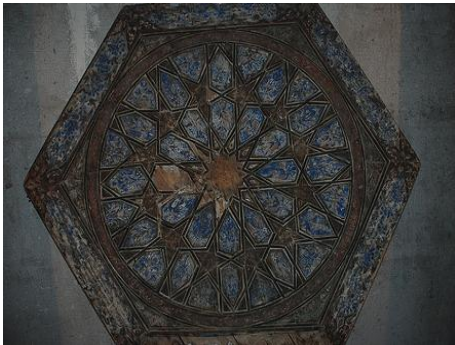
Figure 6. Wood Jointing Ceiling from Konya Ince Minare Museum Konya.
