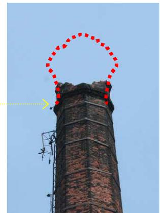
**Figure 3:** Damage extent of the south chimney top portion before and after earthquake [6]
