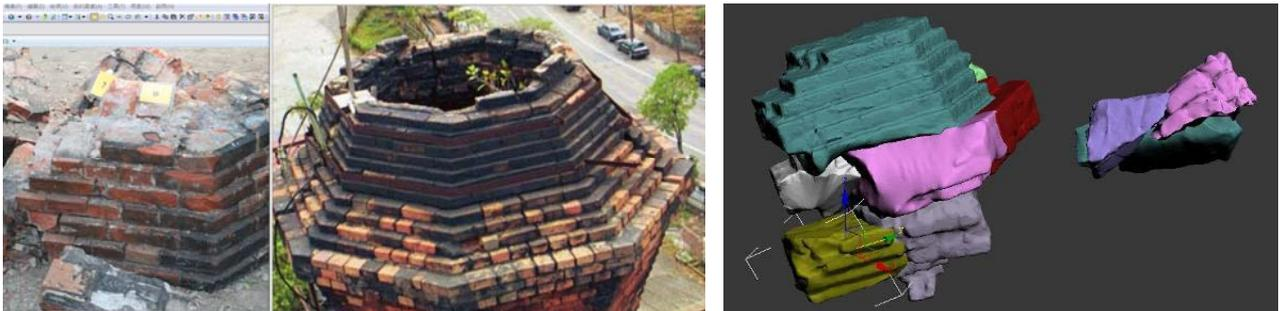
Figure 16: Simulated model of reassembly is achieved by cross-referencing with the existing pictures
