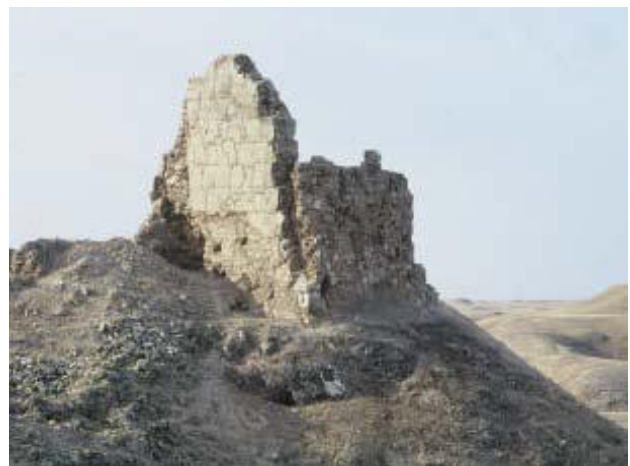
Fig. 6. The still partly standing south-western corner tower of the fort taken from the SW. Photo: Minna Lönnqvist
