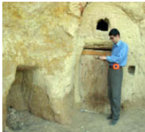
Figure 13. Manual inspection and recording of detail
