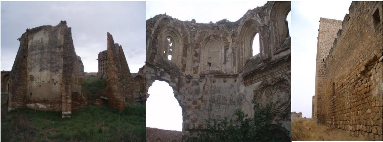
**Figure 1:** 1) Lack of verticality in walls of Chartres of Aniago (Valladolid, Spain). 2) Dangerous vaults in Aniago. 3) External walls in a Spanish Castle (Trigueros del Valle, Valladolid)
