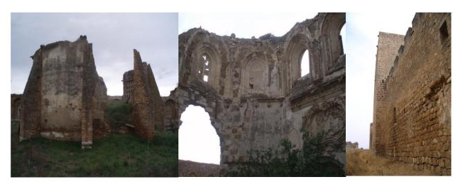
**Figure 1**: 1) Lack of verticality in walls of Chartres of Aniago (Valladolid, Spain). 2) Dangerous vaults in Aniago. 3) External walls in a Spanish Castle (Trigueros del Valle, Valladolid)
