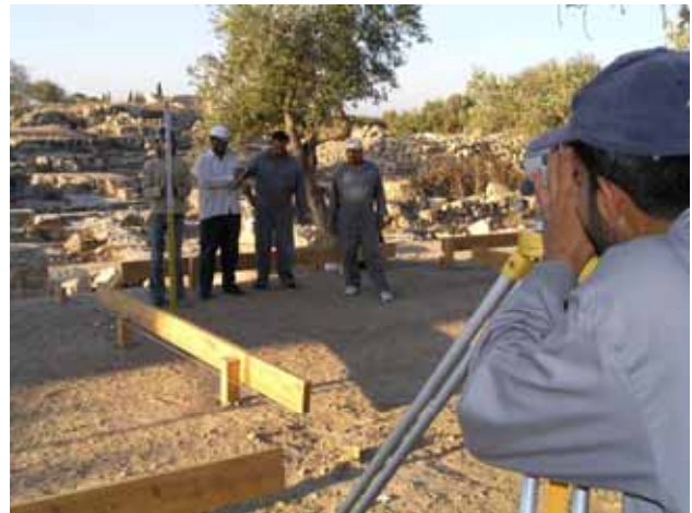
Photo.2 Survey using batter boards
