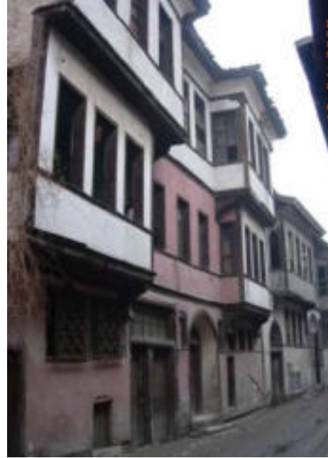
Figure 6. View from the Germiyan Street
