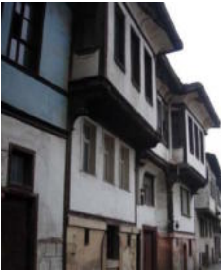
Figure 5. View from the Germiyan Street
