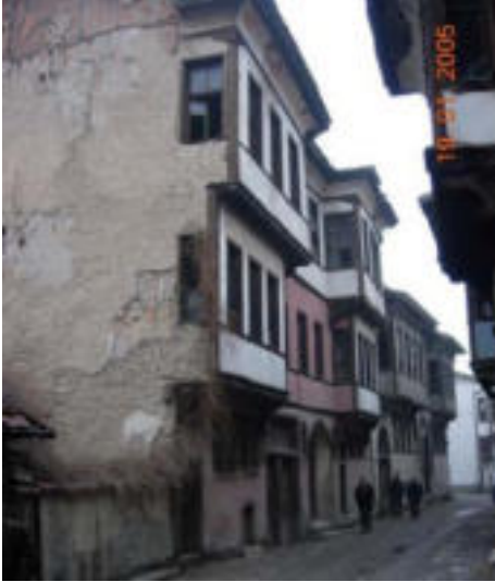
Figure 4. View from the Germiyan Street
