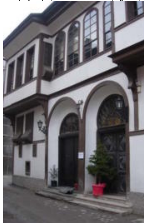
Figure 7. View of the Germiyan Kiosks (restaurant) from Germiyan Street.
